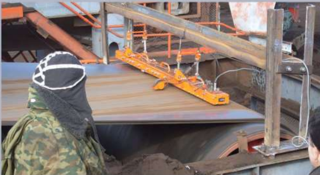
INSPECTION OF CONVEYOR BELTS
