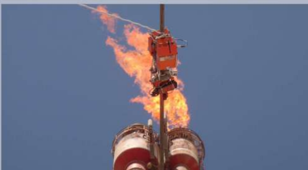
INSPECTION OF FLARE STACK GUY ROPES
