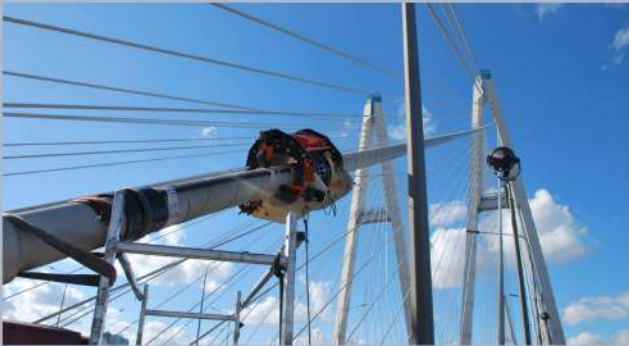
MRT OF BRIDGE CABLES
